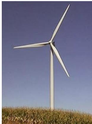
**Gambar 2. 1** Turbin Angin Sumbu Horizontal
