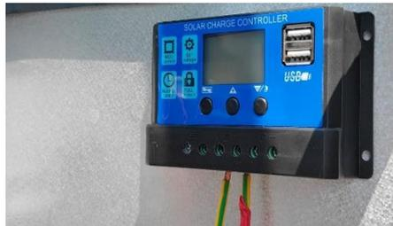
**Gambar 2. 9** Solar Charge Controller
