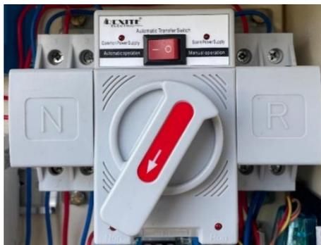
**Gambar 2. 5 Automatic Transfer Switch**
