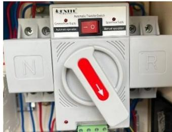
**Gambar 2.6 Automatic Transfer Switch**
