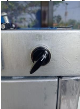
Gambar 2. 4 Selector Switch
