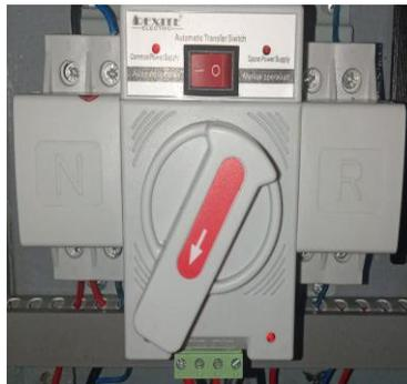
**Gambar 2. 16** Automatic Transfer Switch
