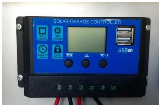
**Gambar 2. 17** Solar Charge Controller
