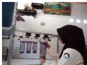
Pemasangan catridge dan housing filter
