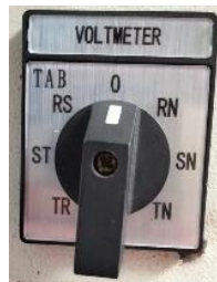
Gambar 2.11 Voltmeter selector switch
