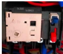
Gambar 2.8 Thermal Overload Relay
