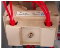
Gambar 2. 12 Current Transformator (CT)
