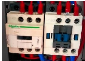
Gambar 2.9 Magnetic Contactor
