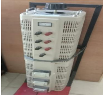
Gambar 2.6 Variable Transformator
