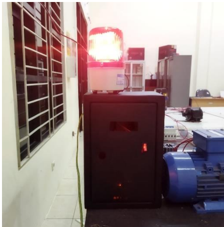
Gambar (B) Perangkat Receiver Saat Ada Emergency
